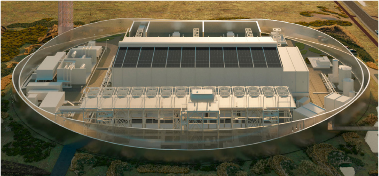
Green-hydrogen factory Holland Hydrogen-1
