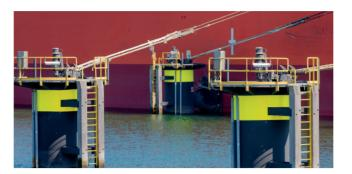
The Port of Rotterdam provides 25 multi-user berths for ship-to-ship transfers throughout the port area. Vessels of any size and any draft can moor at these buoys and dolphins in Rotterdam's sheltered waters for risk-free, continuous and efficient transhipment of all types of dry or liquid cargo, or for repairs, bunkering, cleaning and lay-by.
