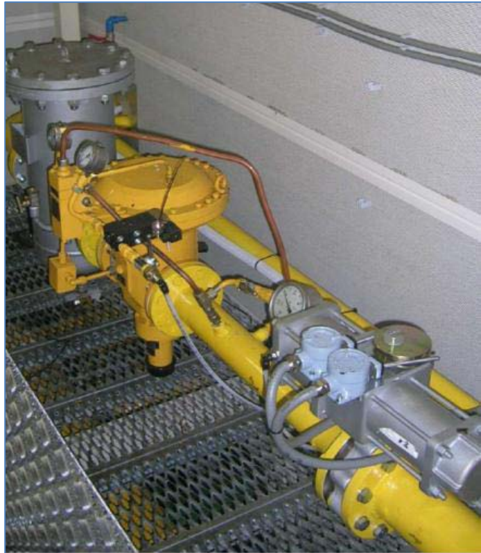
Figure 15. Open GVU. Source: Wärtsilä
