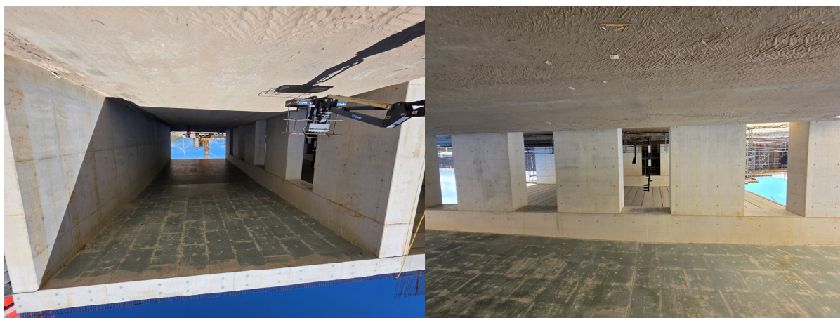
End result after removing formwork
